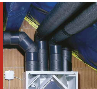
Enormous time saving: IsoPipe®, the insulated duct system.
