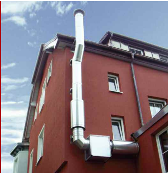
Outdoor installation with wall bracket (accessories).
